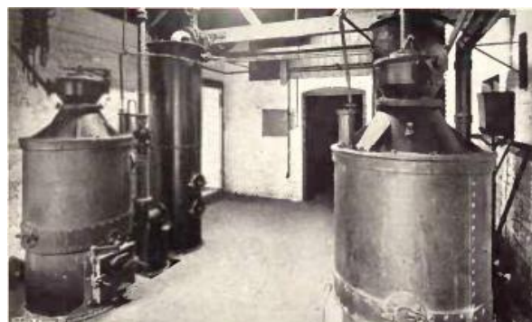
Fig. 7. Suction Gas Producers at Canwell.
